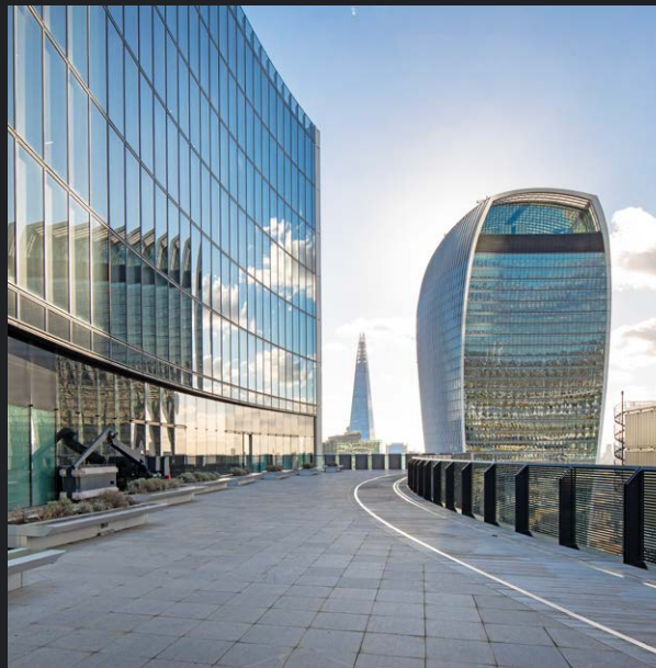
51 Lime Street – 15th Floor Terrace
